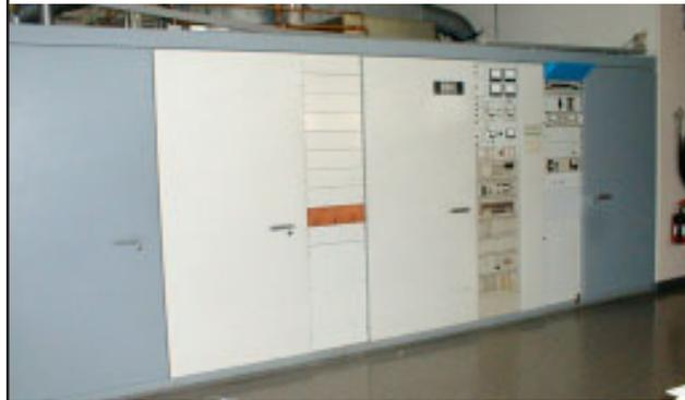
*The 250 KW transmitter ready for broadcasting*
